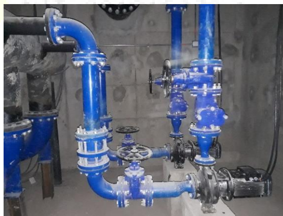
Ilustración 90. Manifold sistema WAS
