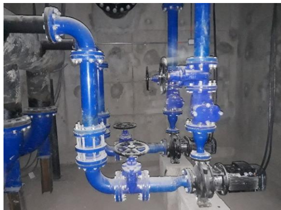
Ilustración 41. Manifold sistema WAS
